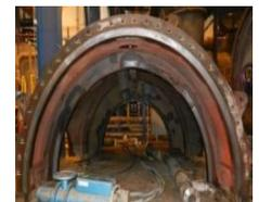
**REPAIRING OF DIFFUSER CASING**
